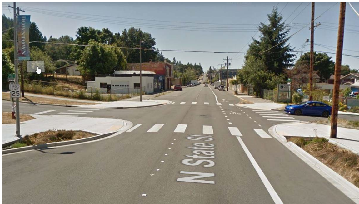
An effectively designed intersection in Bellingham, WA that has curb extensions, ADA ramps, crosswalks and a connection to a nearby trail system.
