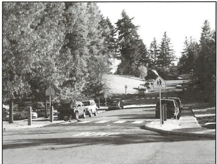
Raised crosswalks, curb extensions, and bollards were installed in this school zone in Bellevue as part of a two-year project to change driver behaviors. Education and enforcement, as well as less expensive signing and pavement markings were also used.
