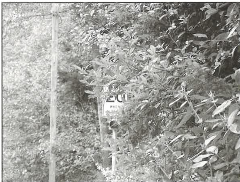
During the annual review, be sure to check that all road signs are clean and not blocked by shrubbery. Contact your public works department or county planning office if needed.
