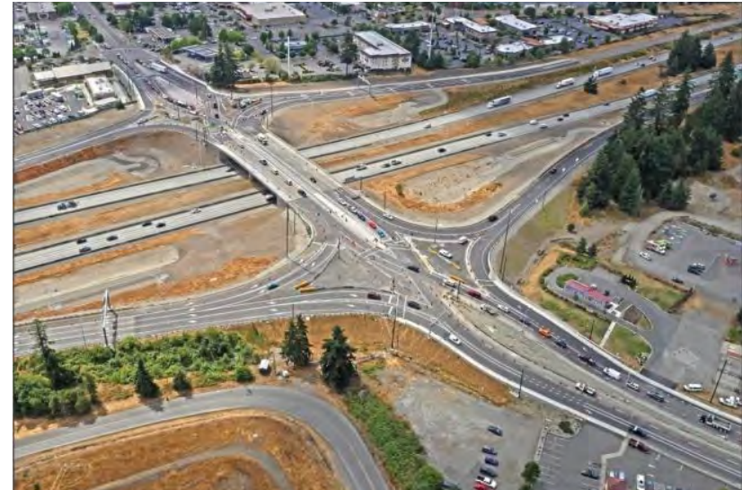
FIGURE 19. DIVERGING DIAMOND INTERCHANGE AT I-5 AND SR-510, LACEY, WA [WSDOT]
