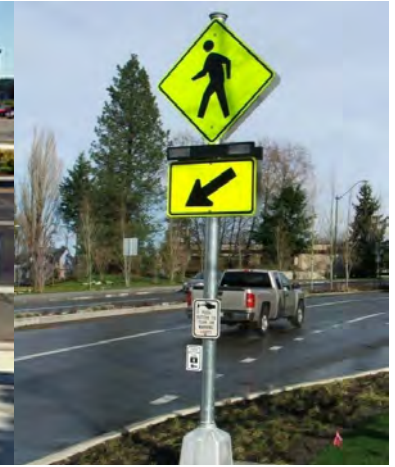
Rectangular Rapid Flashing Beacons
