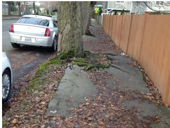
Sidewalk cracked by tree roots, Seattle
