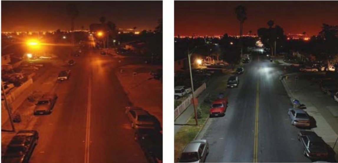
Figure 4: High-Pressure Sodium Lights (left) versus LED Lights (right)
